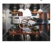
These sensors are designed to be fixed by the case. They may be either vertically or horizontally mounted. The secondary connection is made with a connector. For HBO sensors the primary conductor may be a cable or a bar.
