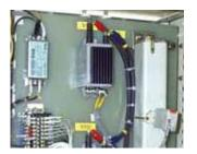
Closed loop Hall effect technology also allows for voltage measurement.
